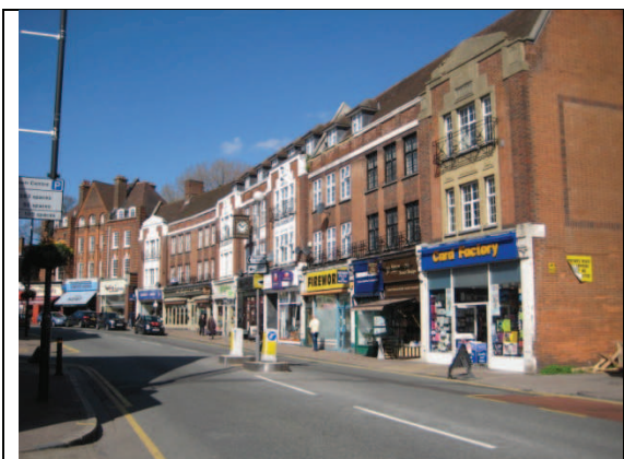
High Street with no 134 in the foreground.
